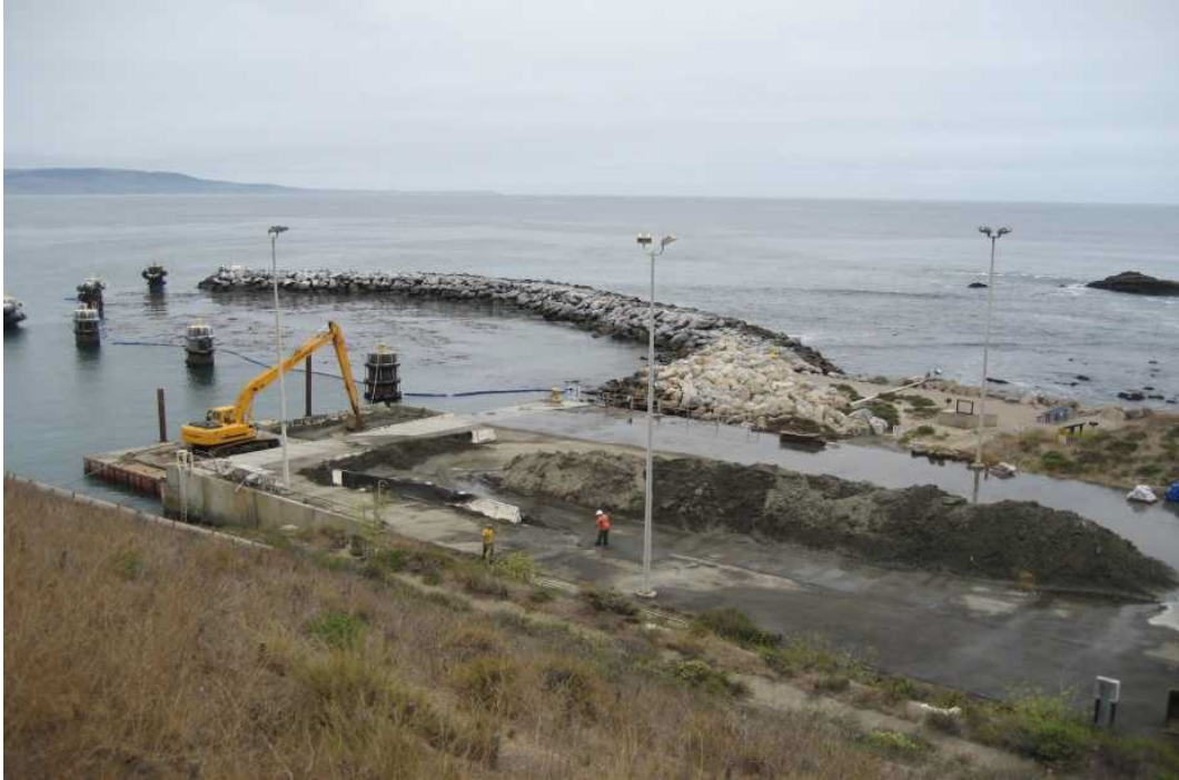
Figure 2-2. Dredging and Sediment Staging with 70-foot Crane
