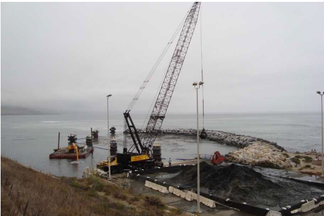
Figure 2-3. Dredging and Sediment Staging with 200-foot Crane
