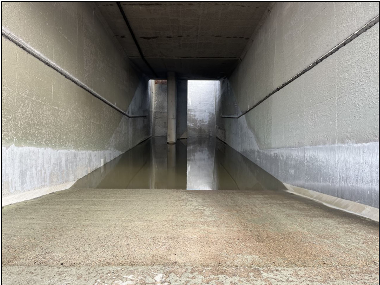
Figure 4.4-8. Flame trench at SLC-6.
