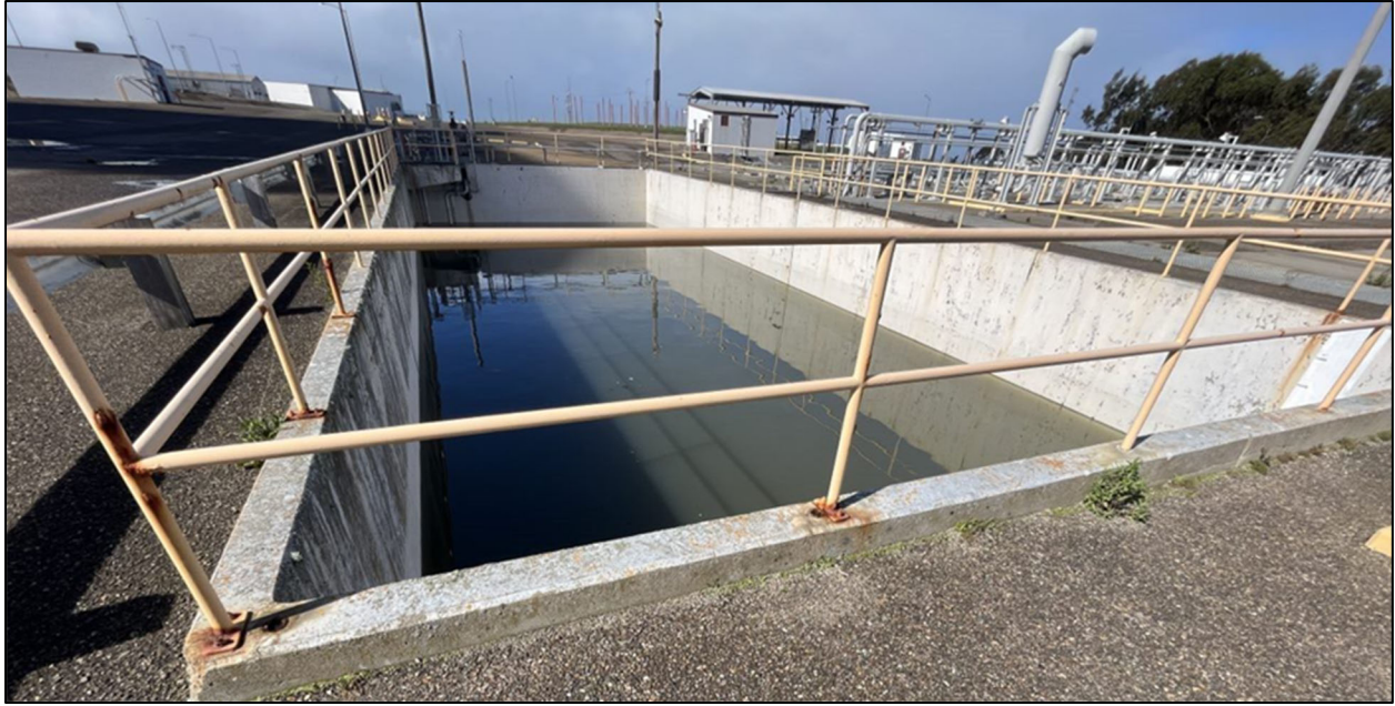
Figure 4.4-7. Vault structure at SLC-6.
