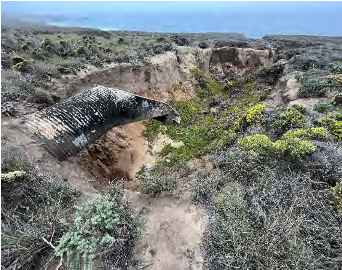
Figure 2-1. Culvert 10 and Channel Degradation at the Culvert 10 Outfall
