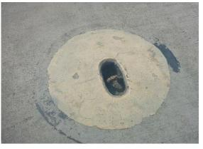
Figure 2-2 Existing Ramp Tie-Down
