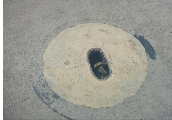
Figure 2-2 Existing Ramp Tie-Down
