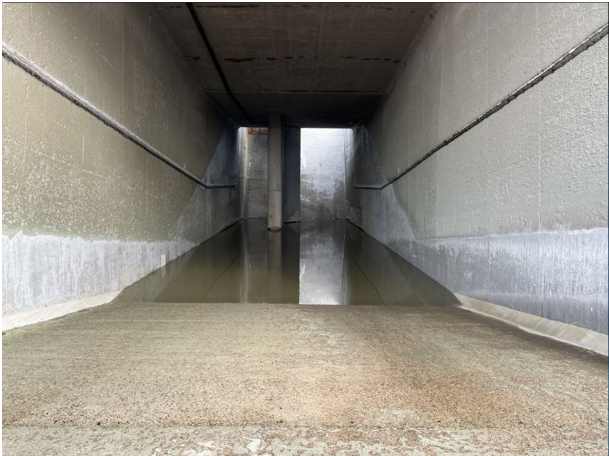
Figure 4.4-5. Flame trench at SLC-6.
