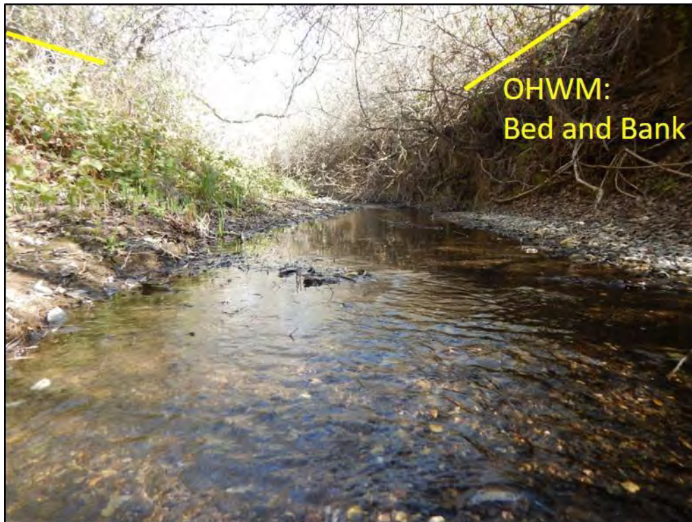
Figure 5-6. Bed and banks of Honda Creek upstream of the culvert intakes.
