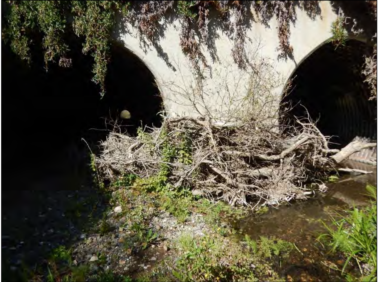
Figure 2-3. Inlet end of the Honda Creek culverts showing trapped debris and sediment.
