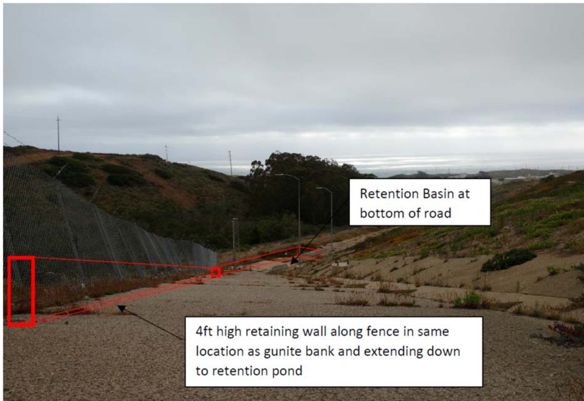
Figure 2-8. Mock-up of Proposed Perimeter Wall on Existing Concrete Apron
