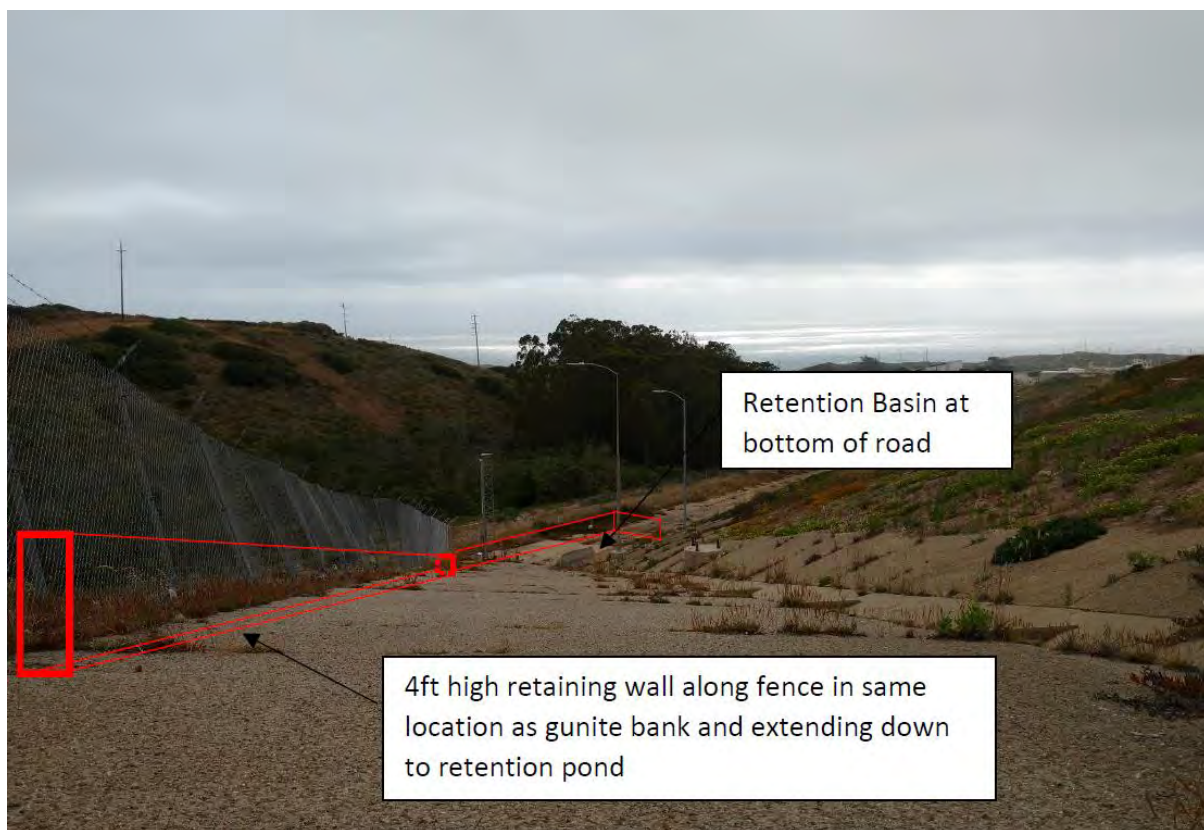
Figure 2-4. Mock-up of Perimeter Wall Design on Existing Concrete Apron
